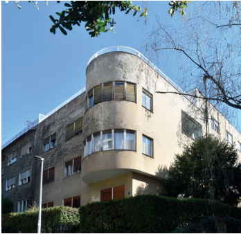
Fig. 11 Moses Lorber, Novakova street n. 21 present view, Zagreb 1935.
